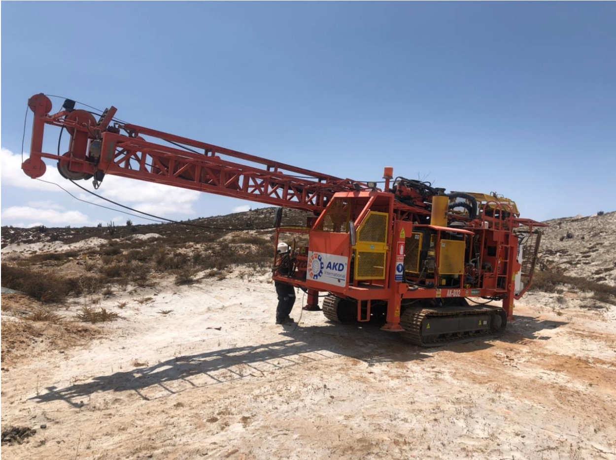
Image 1: Diamond drill rig arriving on site for the start of the Flor de Cobre program.
